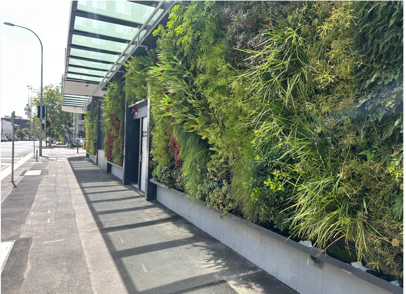
Green wall on private property, Pirie Street
